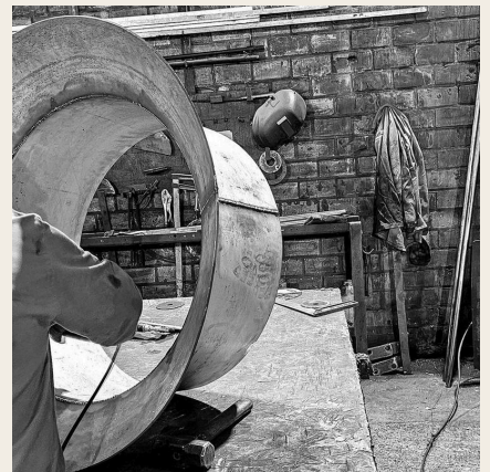
ROLLED SHELL DURING ASSEMBLY
